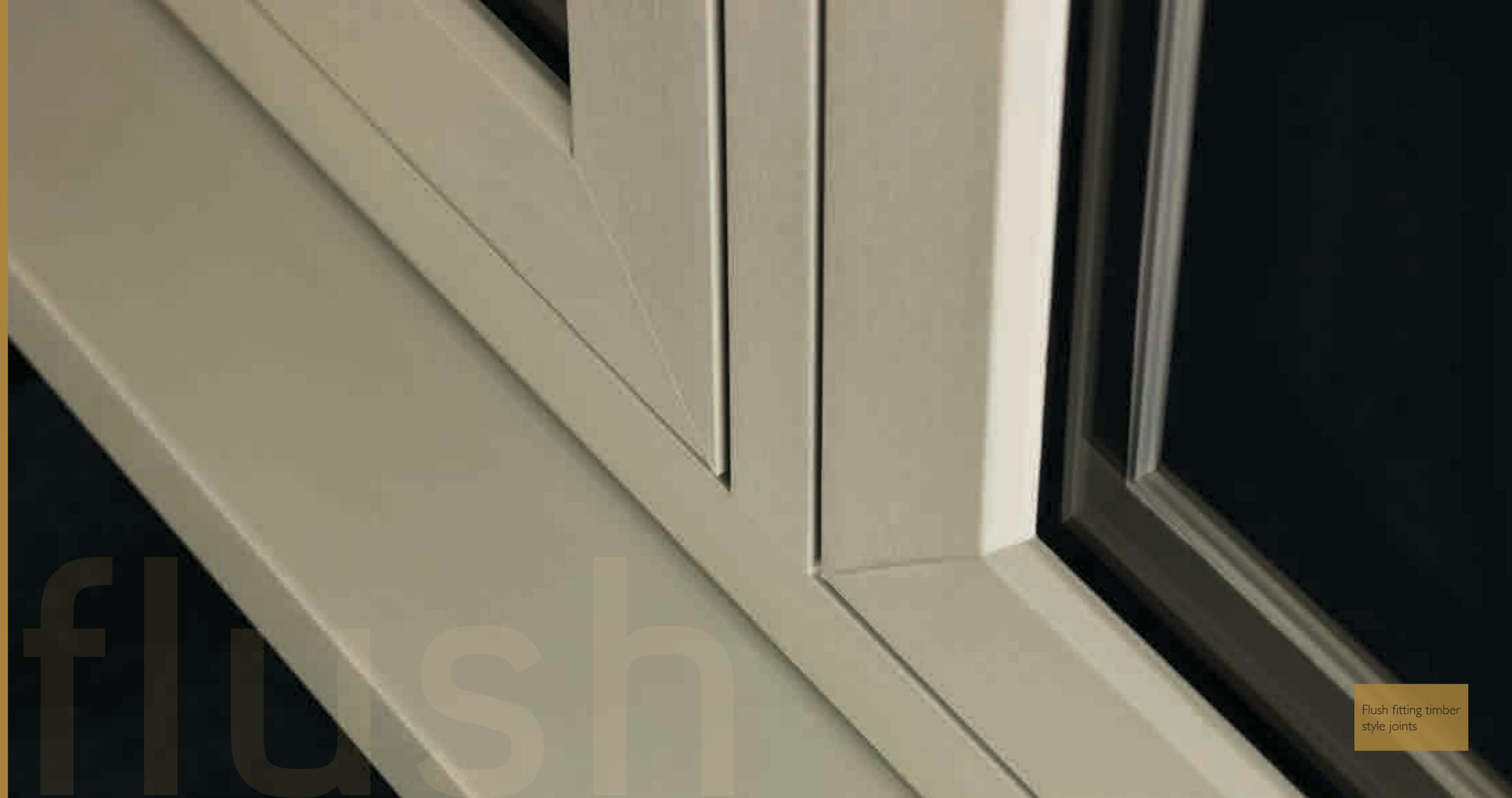
Flush fitting timber style joints
